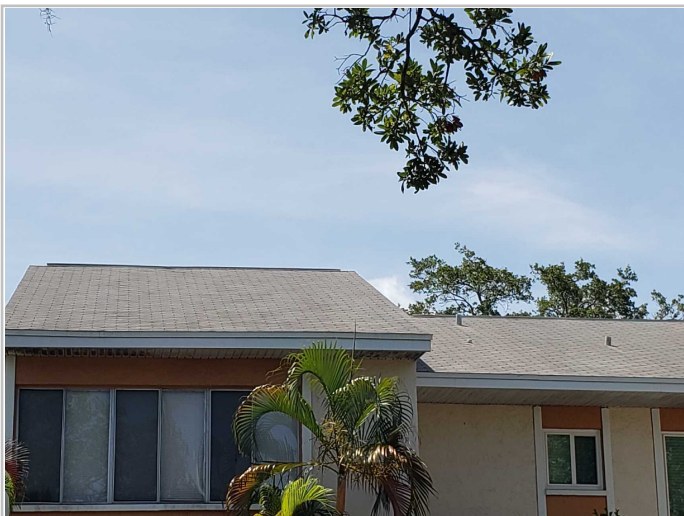
Roof Covering: Asphalt/Fiberglass Shingles
