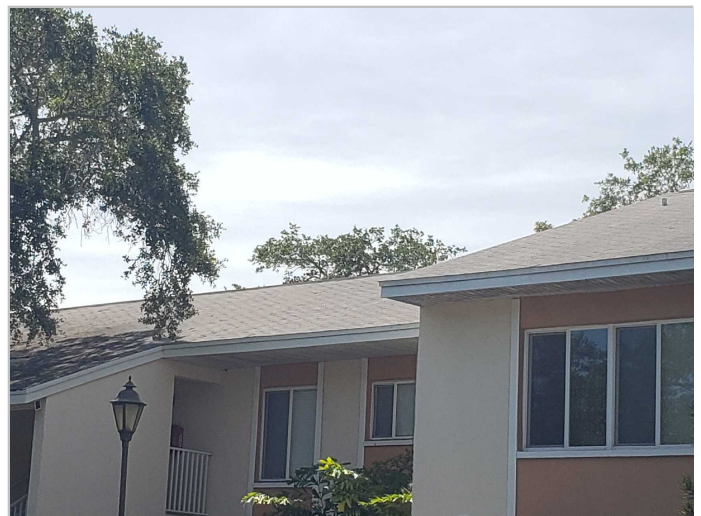
Roof Covering: Asphalt/Fiberglass Shingles
