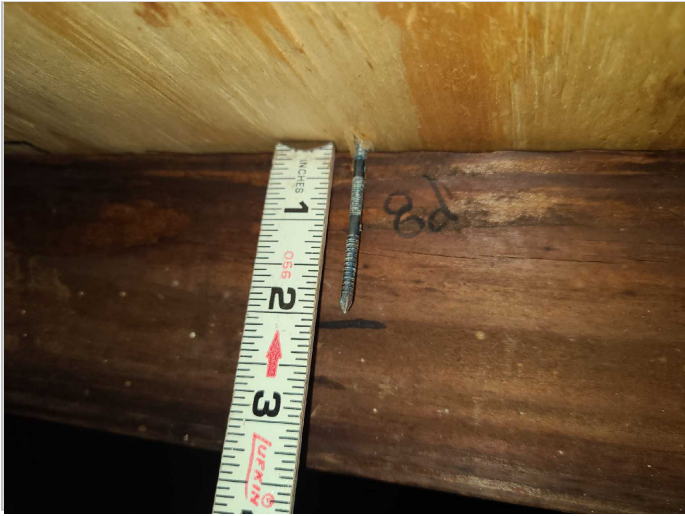
Roof Deck Attachment: 8D Nails
