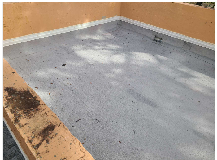
Roof Covering: Modified Bitumen
