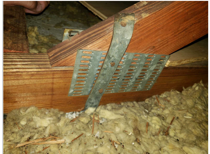
Roof to Wall Attachment: Clips (= or > 3 Nails)
