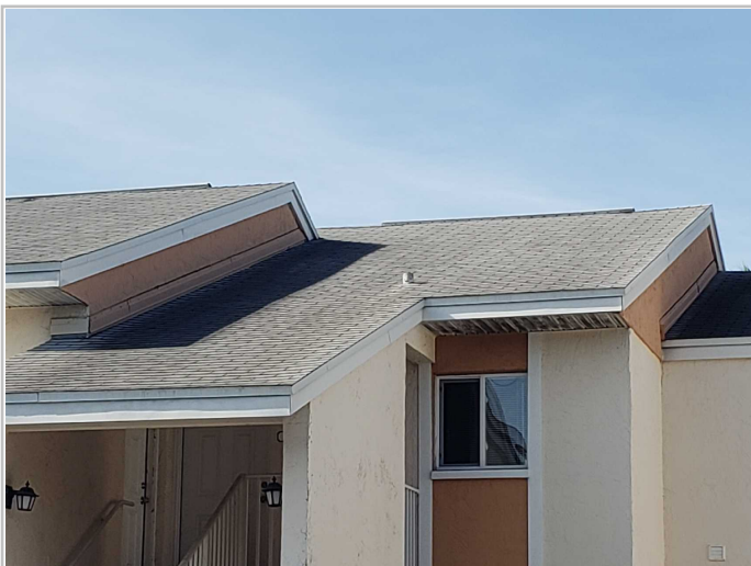
Roof Covering: Asphalt/Fiberglass Shingles
