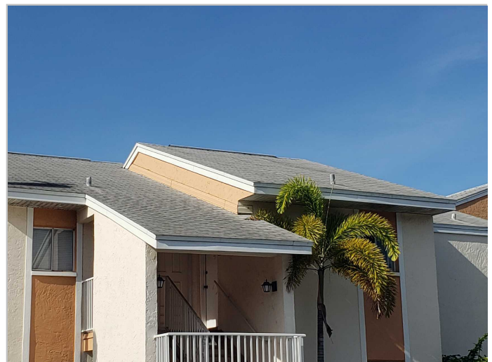
Roof Covering: Asphalt/Fiberglass Shingles
