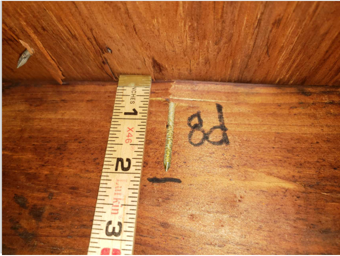
Roof Deck Attachment: 8D Nails
