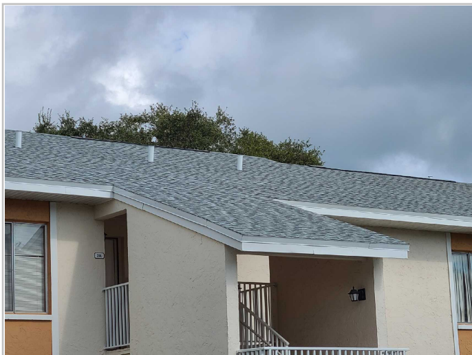
Roof Covering: Asphalt/Fiberglass Shingles
