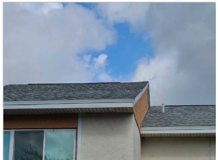
Roof Covering: Asphalt/Fiberglass Shingles
