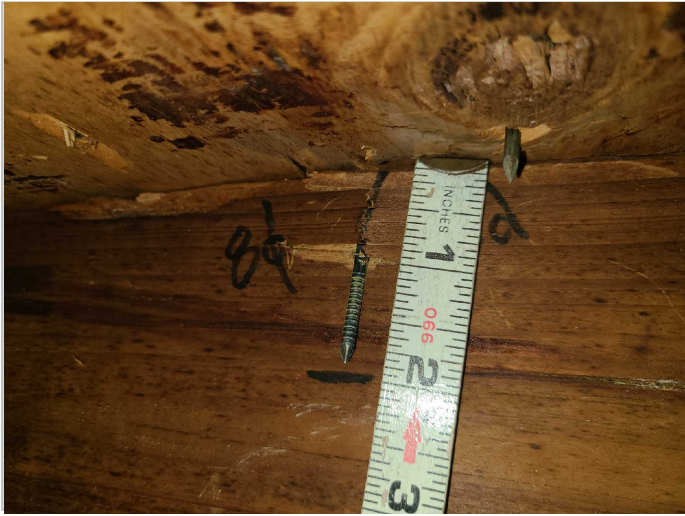
Roof Deck Attachment: 8D Nails
