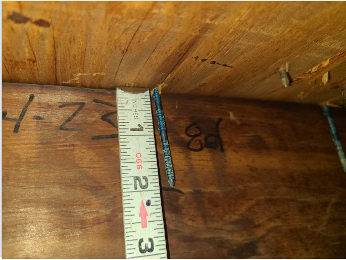
Roof Deck Attachment: 8D Nails
