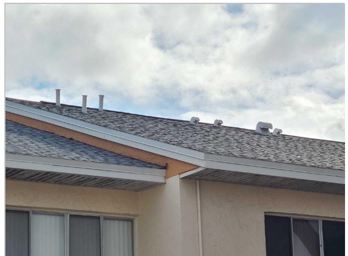
Roof Covering: Asphalt/Fiberglass Shingles
