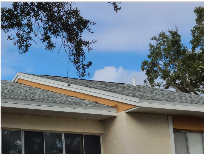
Roof Covering: Asphalt/Fiberglass Shingles
