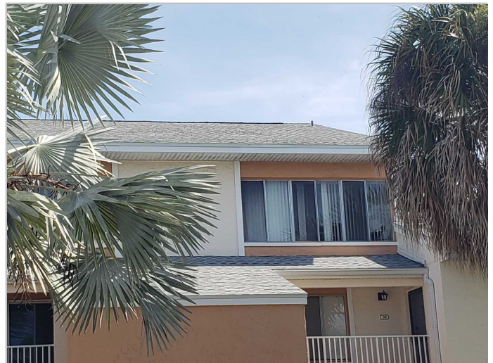
Roof Covering: Asphalt/Fiberglass Shingles
