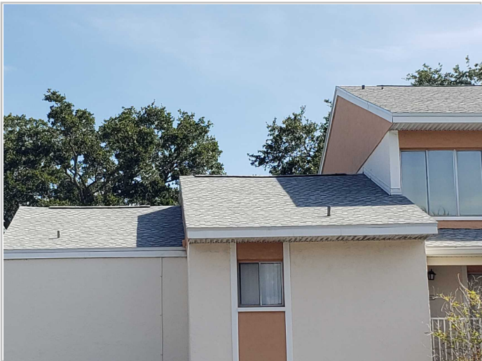
Roof Covering: Asphalt/Fiberglass Shingles
