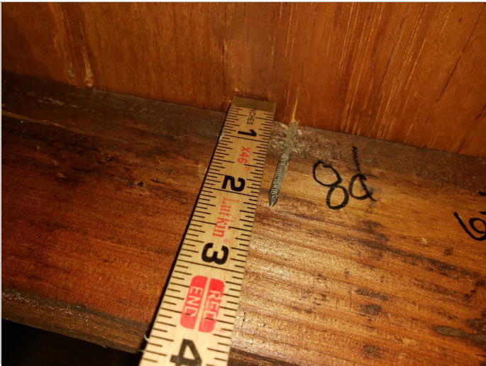
Roof Deck Attachment: 8D Nails
