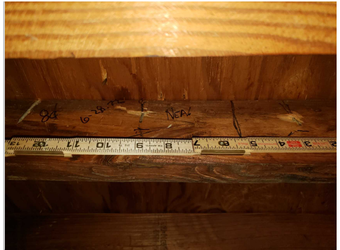
Roof Deck Attachment: 8D Nails (= or < 6" On Center)
