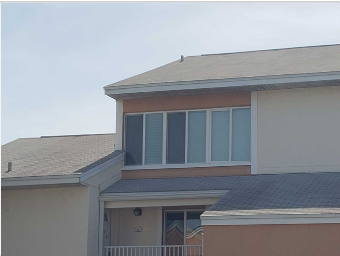
Roof Covering: Asphalt/Fiberglass Shingles
