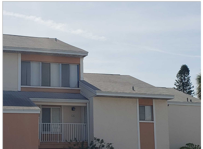
Roof Covering: Asphalt/Fiberglass Shingles
