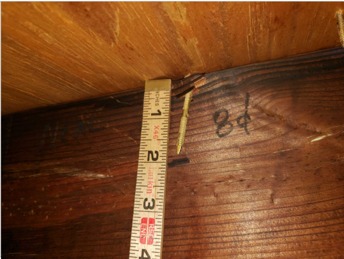
Roof Deck Attachment: 8D Nails
