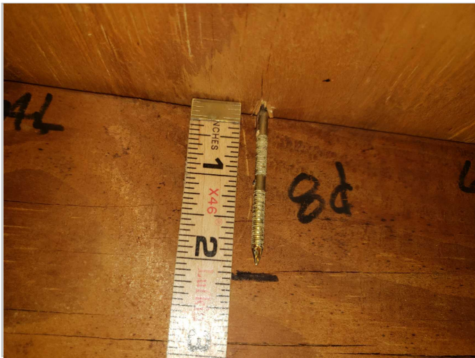
Roof Deck Attachment: 8D Nails
