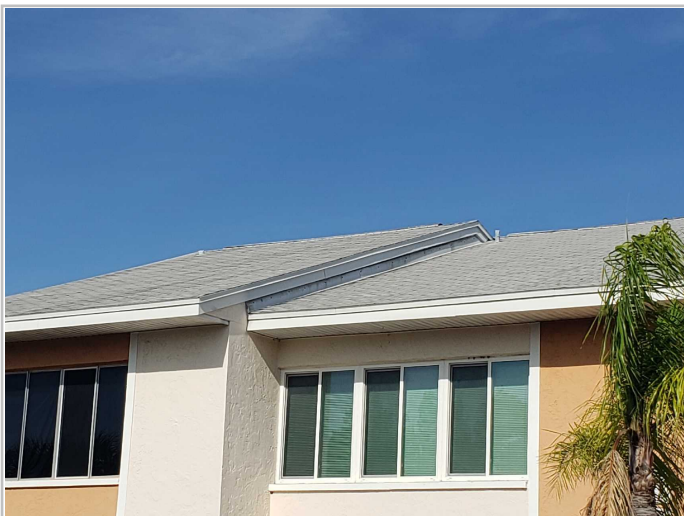
Roof Covering: Asphalt/Fiberglass Shingles
