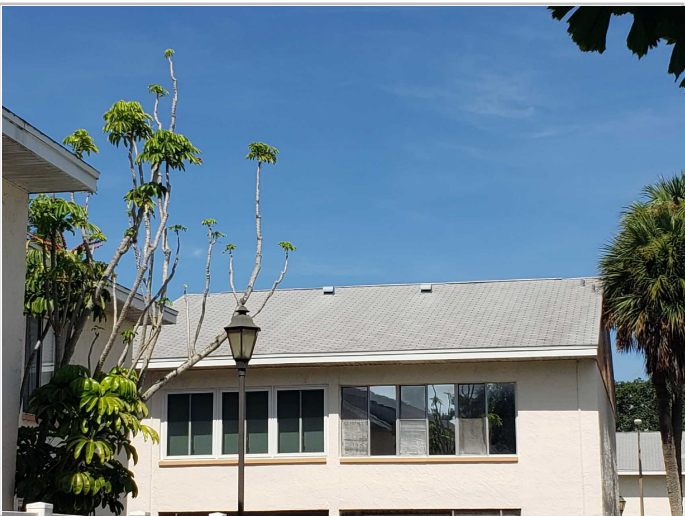
Roof Covering: Asphalt/Fiberglass Shingles
