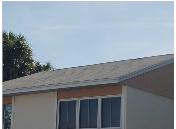
Roof Covering: Asphalt/Fiberglass Shingles
