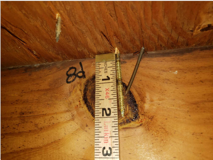
Roof Deck Attachment: 8D Nails
