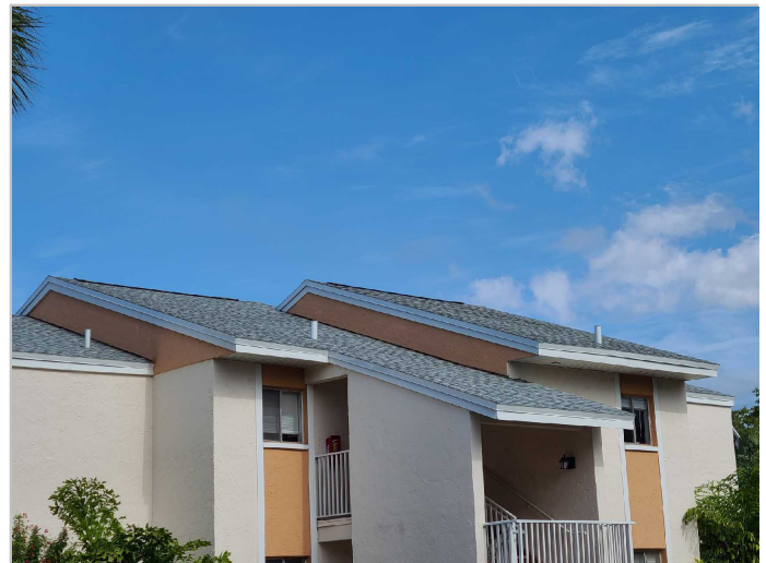
Roof Covering: Asphalt/Fiberglass Shingles
