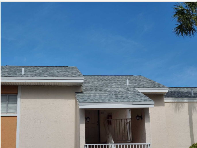
Roof Covering: Asphalt/Fiberglass Shingles
