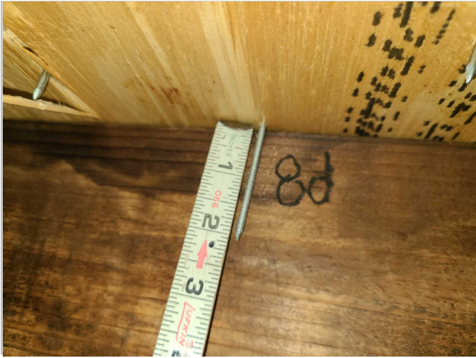
Roof Deck Attachment: 8D Nails
