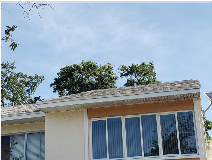
Roof Covering: Asphalt/Fiberglass Shingles
