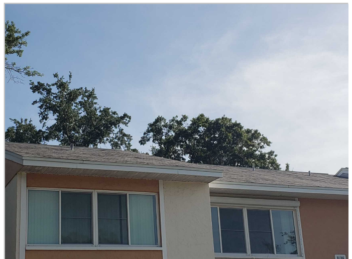
Roof Covering: Asphalt/Fiberglass Shingles
