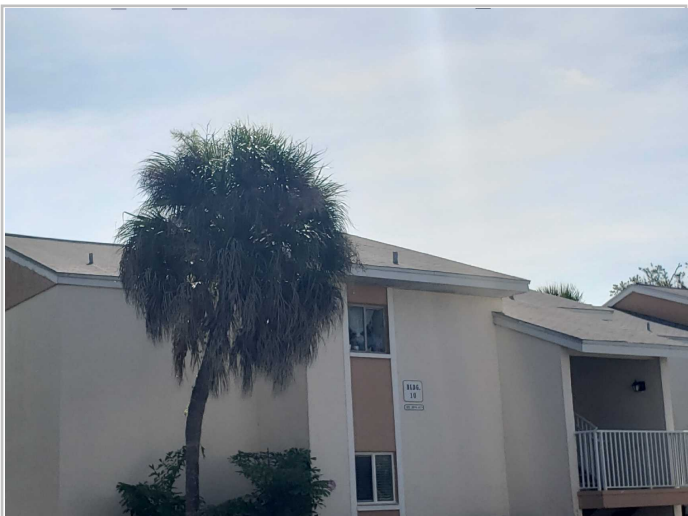
Roof Covering: Asphalt/Fiberglass Shingles
