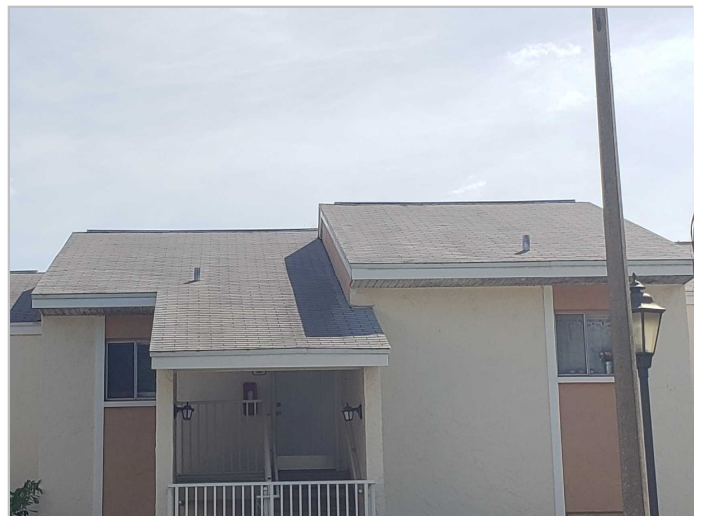
Roof Covering: Asphalt/Fiberglass Shingles
