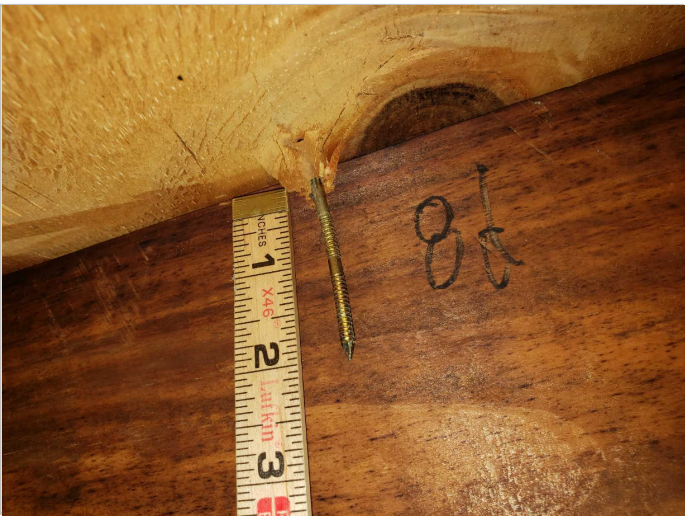
Roof Deck Attachment: 8D Nails
