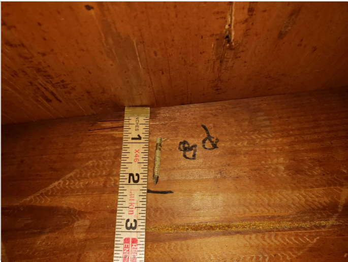
Roof Deck Attachment: 8D Nails
