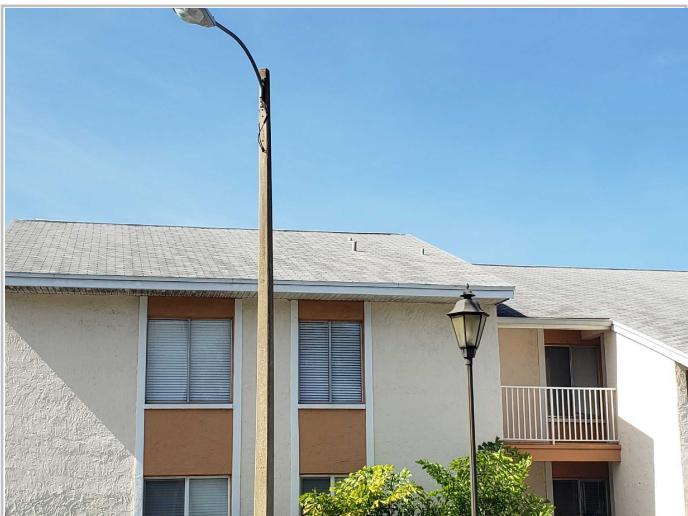
Roof Covering: Asphalt/Fiberglass Shingles
