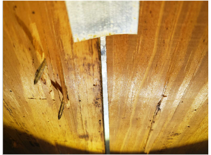
No Secondary Water Resistance (SWR)
