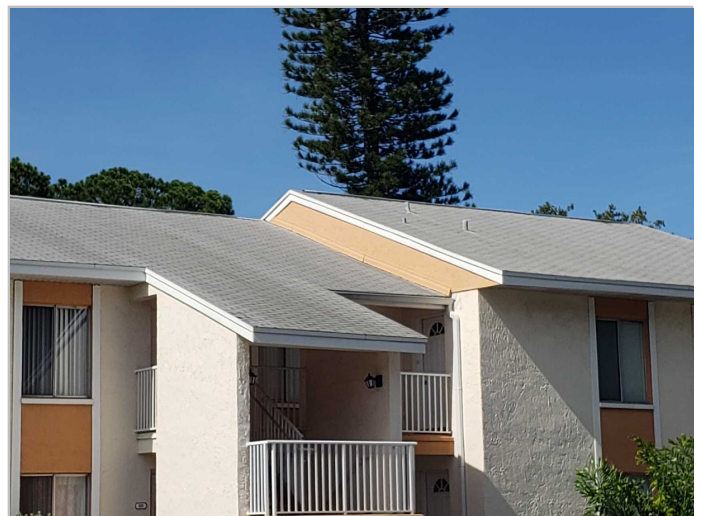
Roof Covering: Asphalt/Fiberglass Shingles
