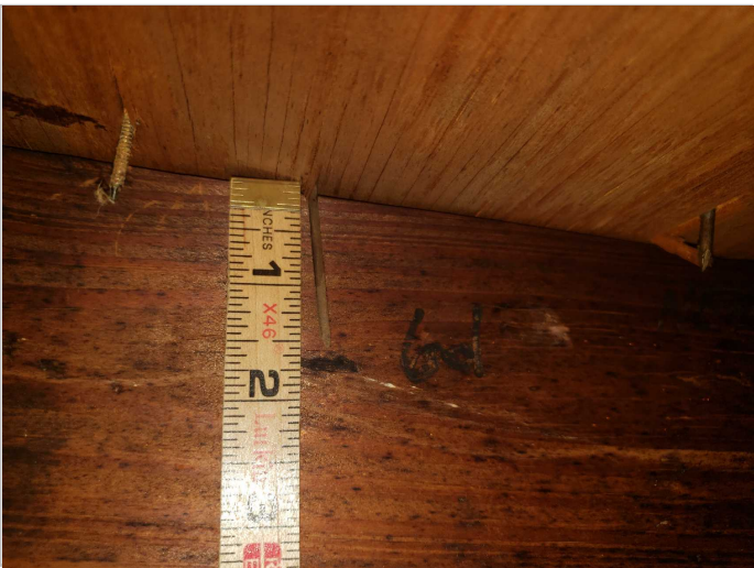
Roof Deck Attachment: 6D Nails
