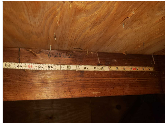
Roof Deck Attachment: 6D Nails
