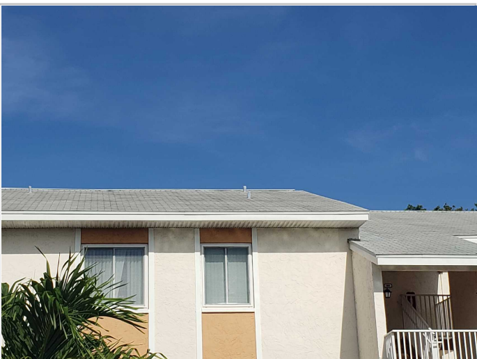
Roof Covering: Asphalt/Fiberglass Shingles
