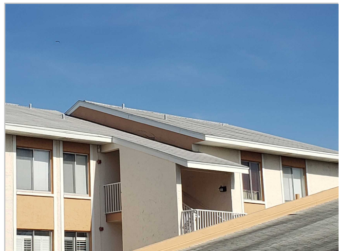
Roof Covering: Asphalt/Fiberglass Shingles
