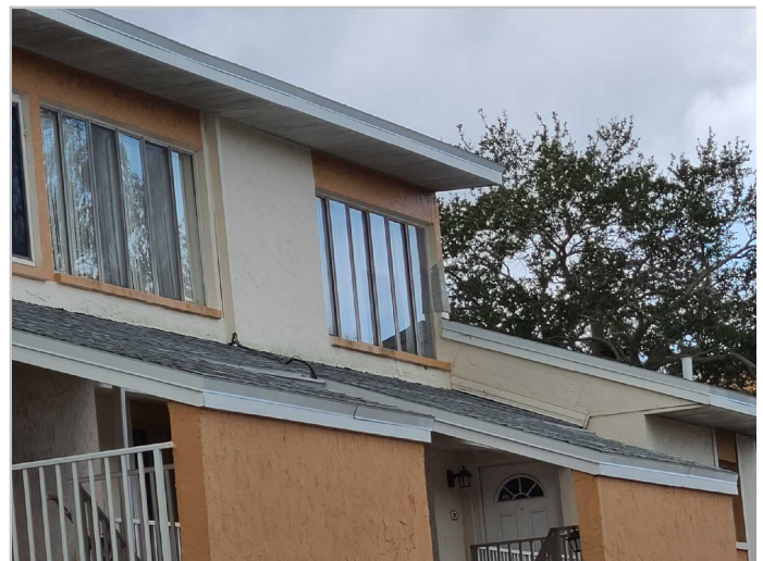
Roof Covering: Asphalt/Fiberglass Shingles
