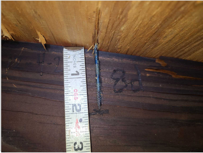
Roof Deck Attachment: 8D Nails
