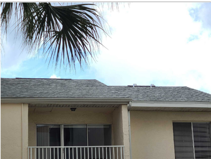
Roof Covering: Asphalt/Fiberglass Shingles
